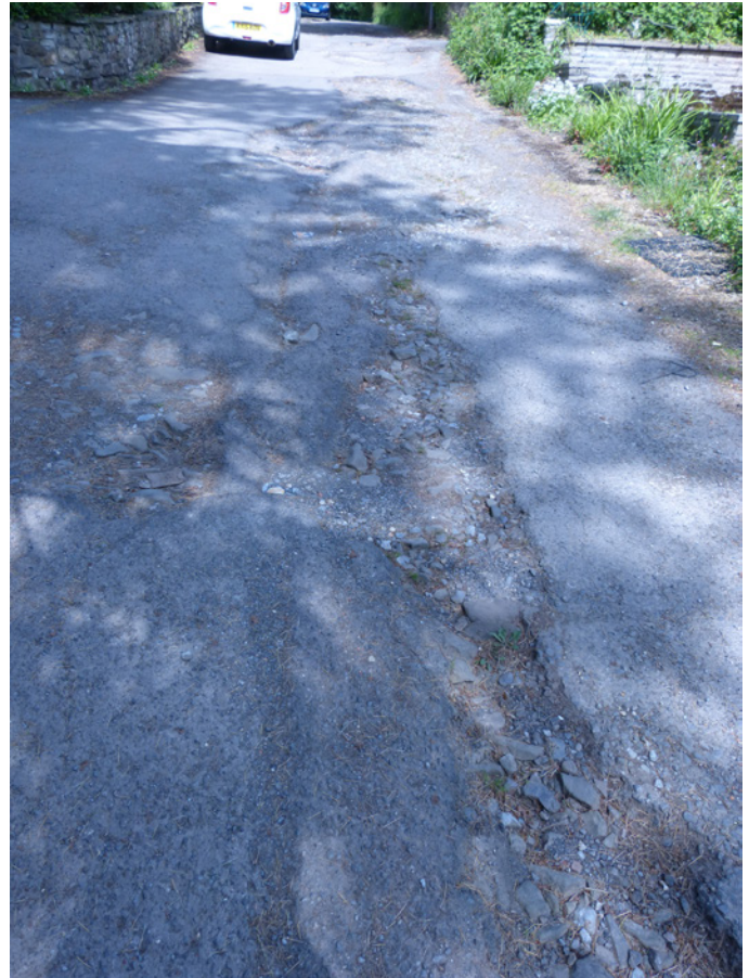
Photograph 14: An area of failing road surface, which will become progressively worse if left untreated
