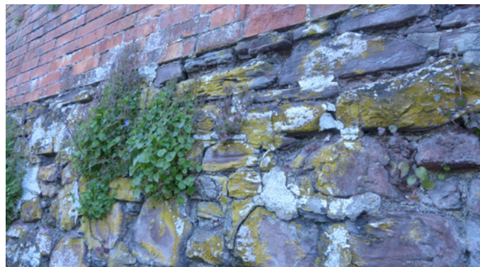
Photograph 15: Vegetation growth, failing pointing and deteriorating stonework on the Fields Road boundary wall
