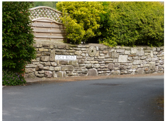
Photograph 17: Re-used masonry in a boundary wall, including a millstone and squared blocks which are likely to have been prepared for a higher-status structure given the skill and time required to finish stone to this standard
