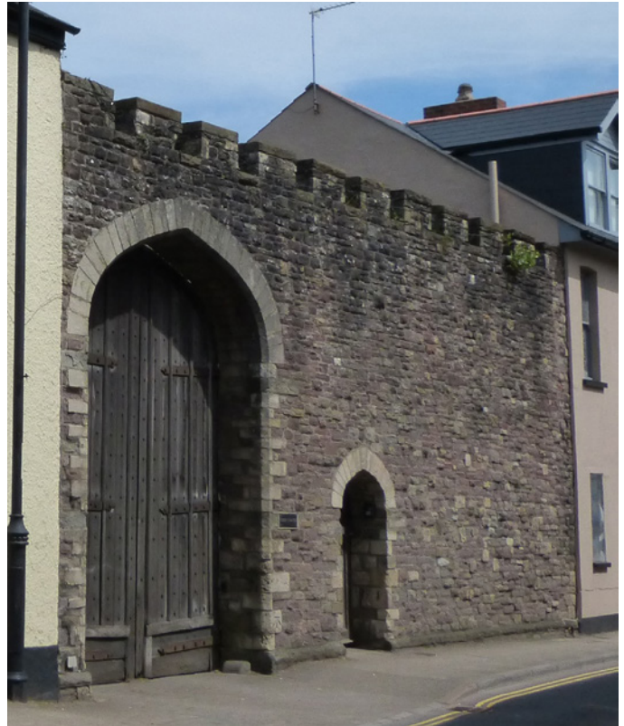
Photograph 16: A section of pennant stone wall with battlements, showcasing a local building material and contributing to the militaristic character of the central section of the High Street
