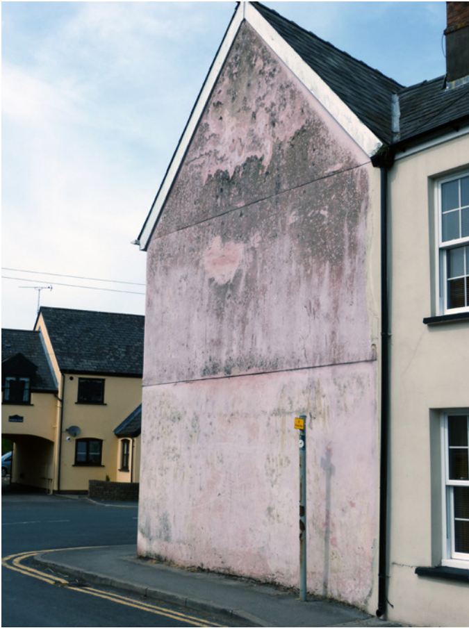
Photograph 24: External mould on an exposed gable end wall
