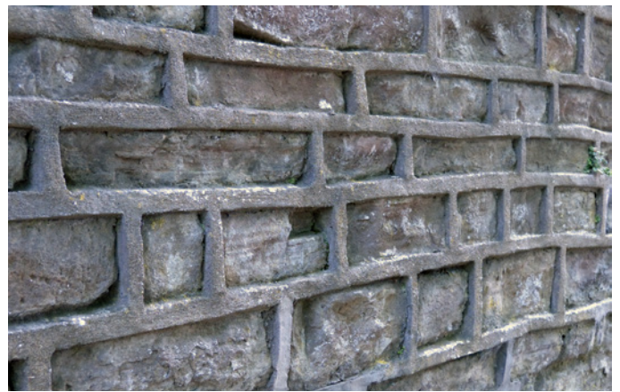
Photograph 26: Extreme ribbon pointing on Castle Lane, which is detrimental to the condition of the stone
