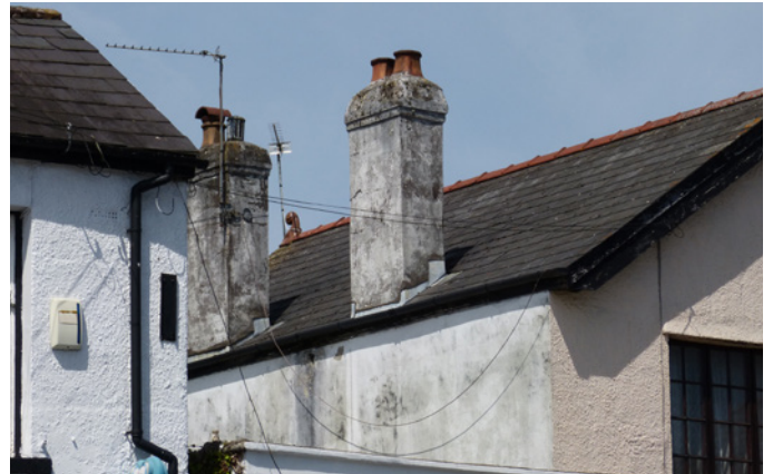
Photograph 25: Mould and algal growth on a chimneystack
