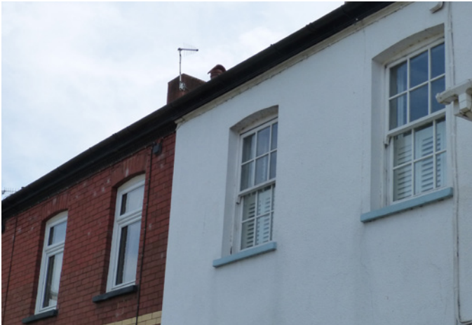
Photograph 29: Traditional sash windows on the right and inappropriate modern replacements on the left
