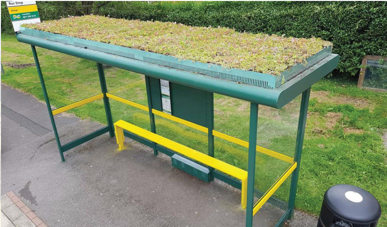
Retrospectively fitted and refurbished green roof shelter
