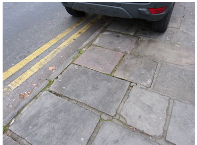
Photograph 22: Loose pavement stones due to cars mounting the kerb to park in undesignated spaces
