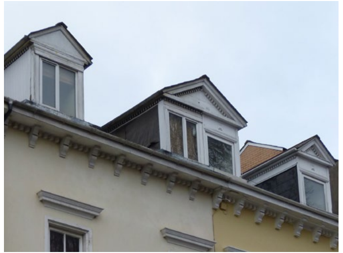
Photograph 29: Replacement dormer window frames in mismatched and inappropriate styles
