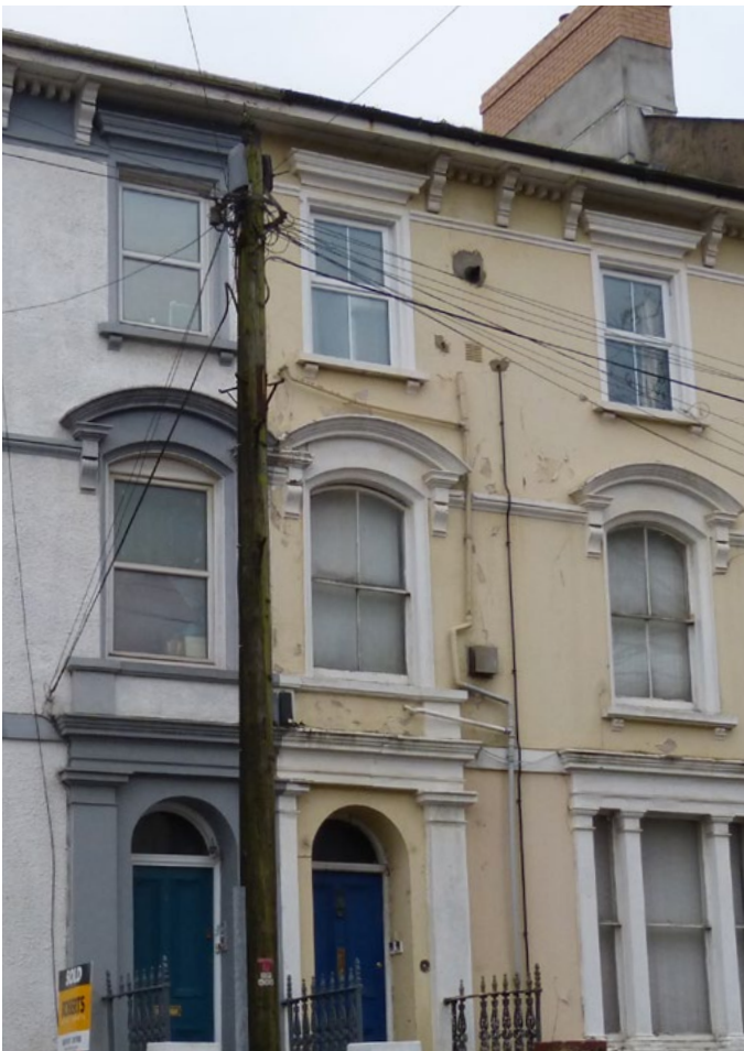
Photograph 30: Flaking paint, external pipework and detracting telephone wires
