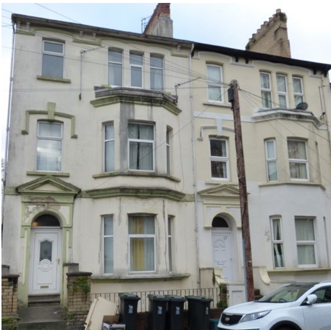
Photograph 18: Staining and flaking paint
