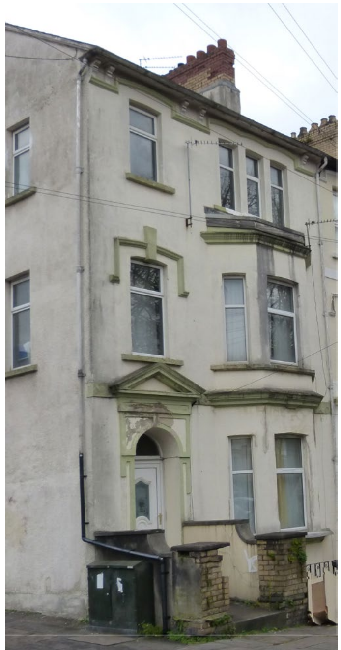
Photograph 19: Stained render and damaged brick piers
